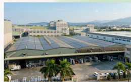
Yunlin Zhuwei Plant
